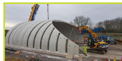
Installation of the green bridge to carry a bridleway over the new link road.
