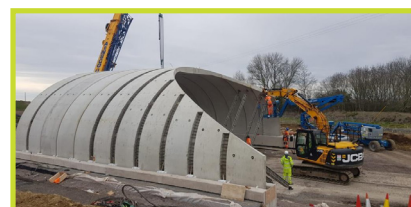
Installation of the green bridge to carry a brideway over the new link road.
