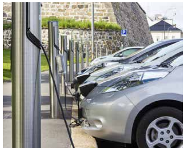
Integrated EV charging points.
