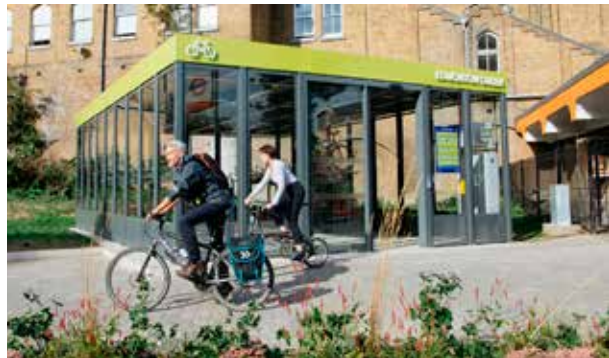
Sheltered bicycle storage.
