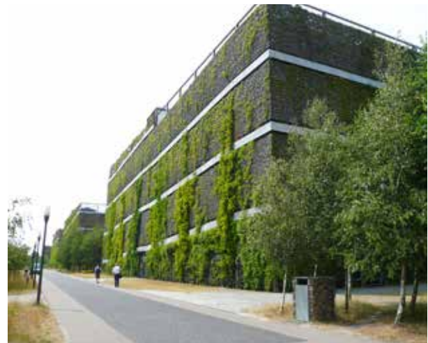
Decked and screened parking areas provide an efficient and attractive means of housing car parking.
