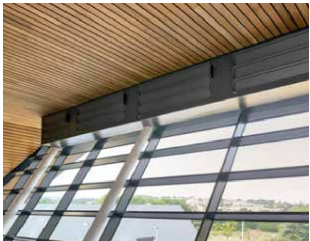
Natural ventilation modules allied with an angled building overhang to mitigate impact of summer solar gain, Exeter Science Park.
